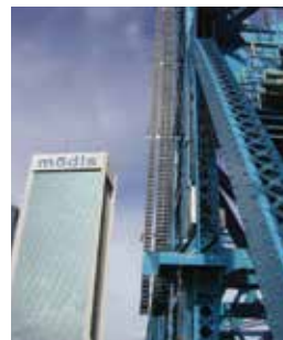
This cable carrier is installed on a vertical lift bridge.
